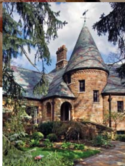
The palatial Baxter-Chumley house in Elm Heights is faced with sandstone from St. Meinrad, Indiana, has limestone details—window sills, steps, benches, and lions—and a slate roof and walkway. The beautifully landscaped yard, maintained mostly by Beth, has recovered nicely from the spring’s cold snap.
