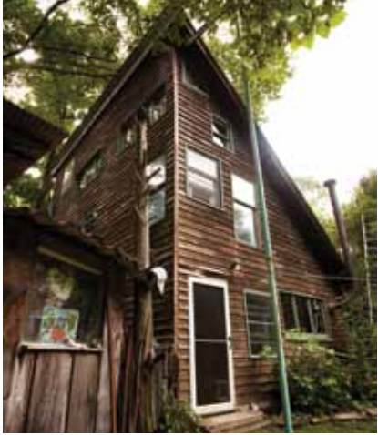
The architecture of this house reflects its passive solar design, which maximizes southern exposure. The siding is western red cedar, which although new, had been discarded or left over from some other job. No piece is longer than four feet, making the boards impractical for a commercial builder.
