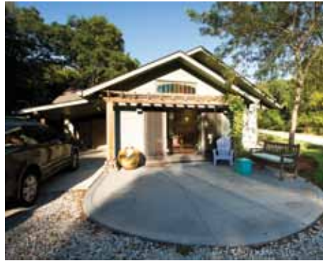
Beebe designed a welcoming front entrance with a patio shaded by a honey locust tree. Instead of leaving the concrete plain, she had it stamped decoratively using a pattern she cut out of rubber entry door matting from a department store.
