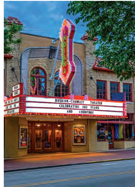
The grant, along with a 30% match from the City of Bloomington, will fund a new HVAC system, a rooftop solar photovoltaic system, and a state-of-the-art solar "battery." Photo by Rodney Margison
