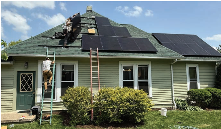
MPI Solar installed 20 solar panels to Bloom's roof in May. Photo by Rodney Margison
