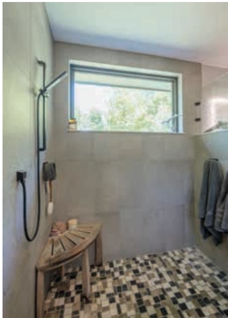
Awning-style windows allow for airflow and natural light while maintaining privacy within the shower space.
